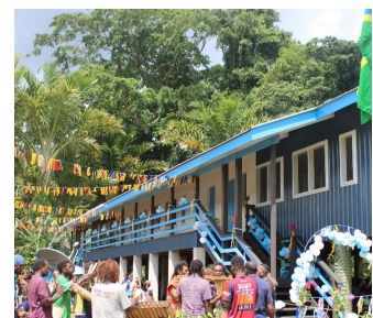
The new classrooms at Manawai Community High School funded by Australia
