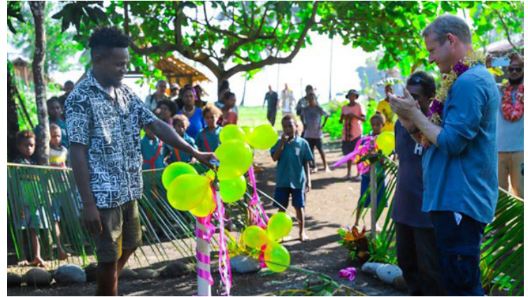
Australian High Commissioner His Excellency Rod Hilton opening the new water source facility in Mwanihuki, Central Makira Constituency, funded through the Solomon Islands – Australia Community Partnerships grants
