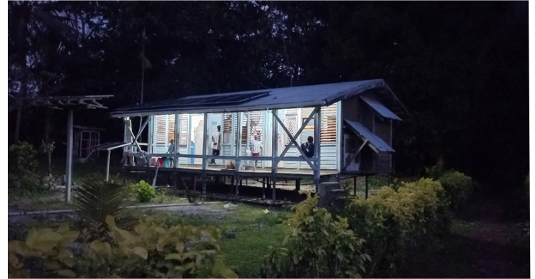
Nuoba Clinic in Temotu Nende now has solar-powered electricity for the first time ever thanks to SBD 164,000 in funding from Australia
